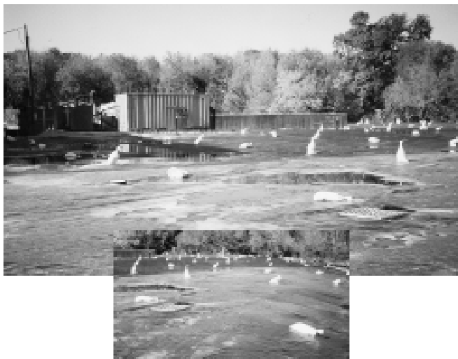
Air Sparging/Soil Vapor Extraction remediation in process
