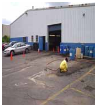
The treatment of a waste oil release to the soil and groundwater at an automotive dealership with Fenton's Reagent
