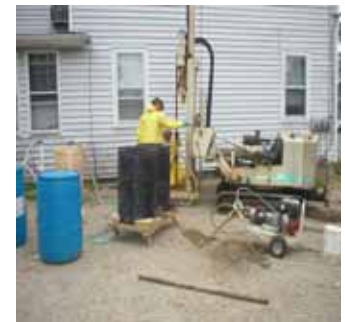
Treatment of soil located below the foundation of a home
