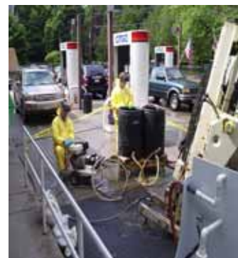
High pressure Geoprobe groundwater treatment at an active gas station
