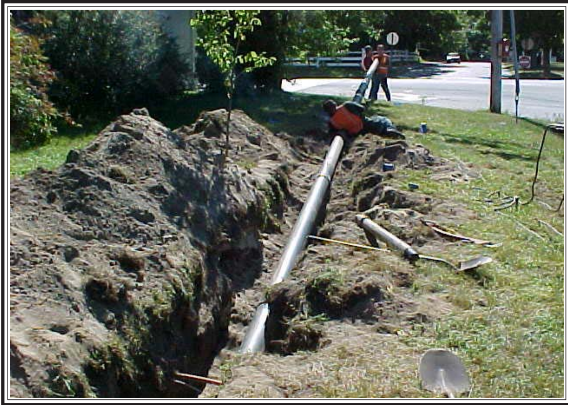
Figure 2, Sewer Pipe Installation
